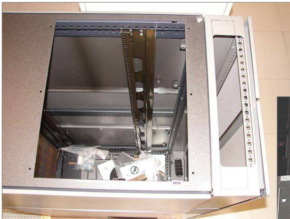
Top Panel After Replacement
